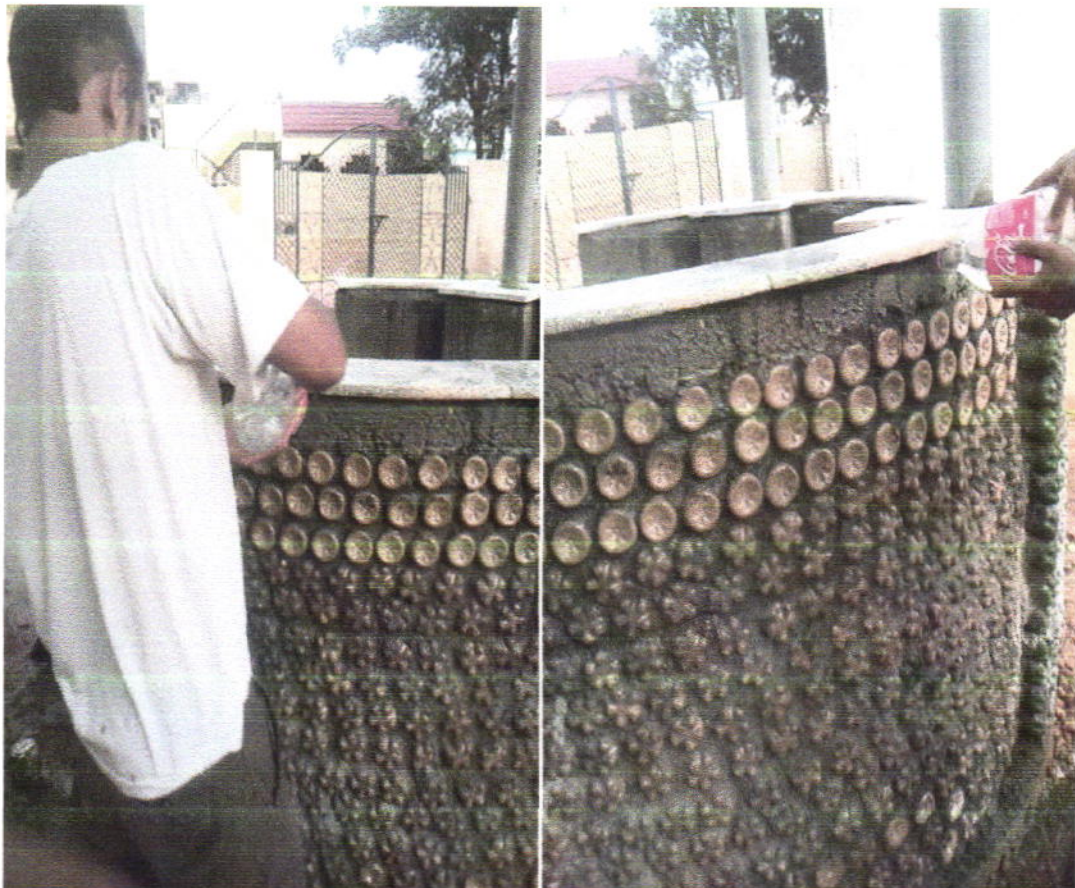
Fig 7.9.1: Curing of the structure
