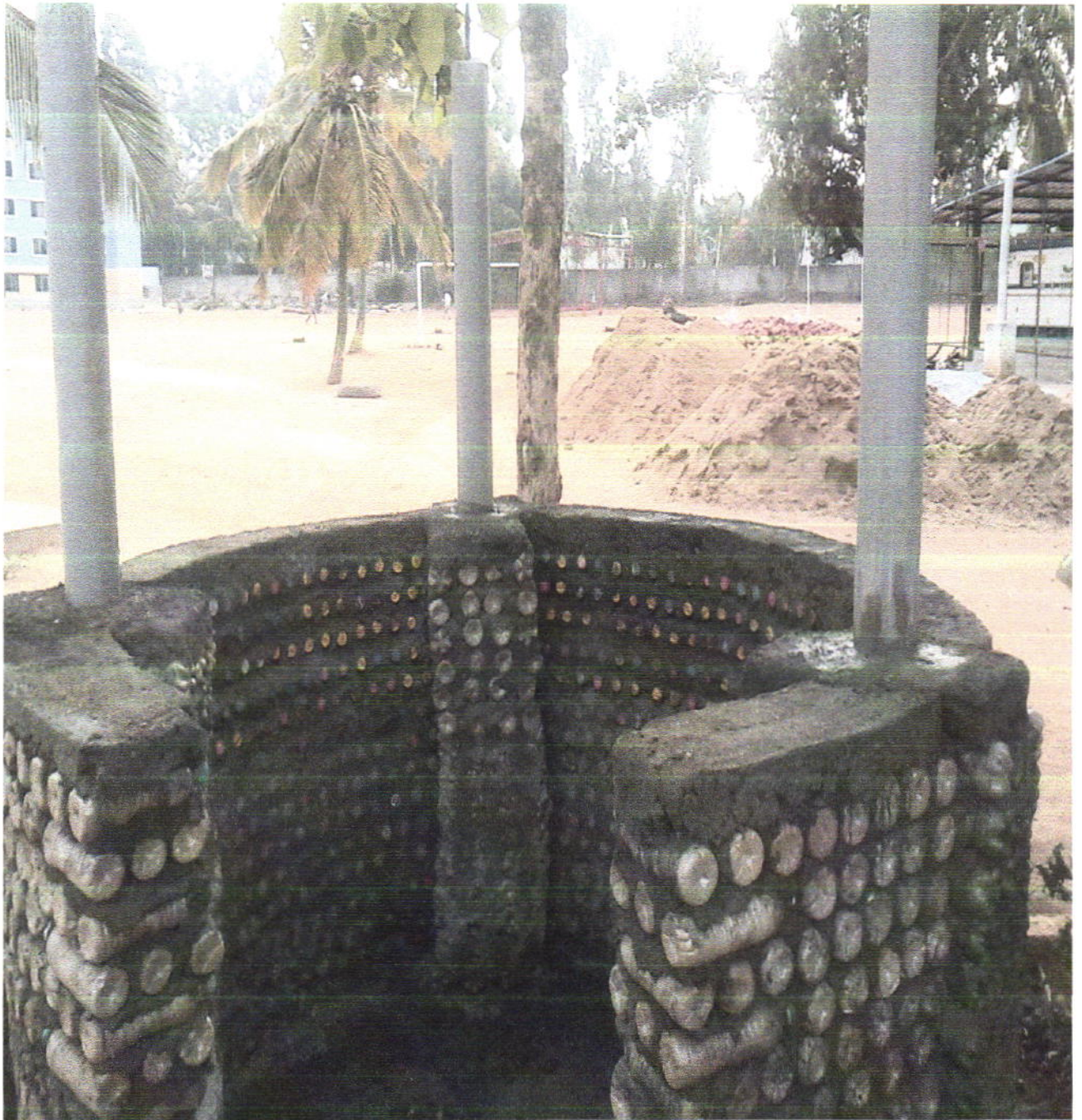
Fig 7.6: Wall built up using plastics
