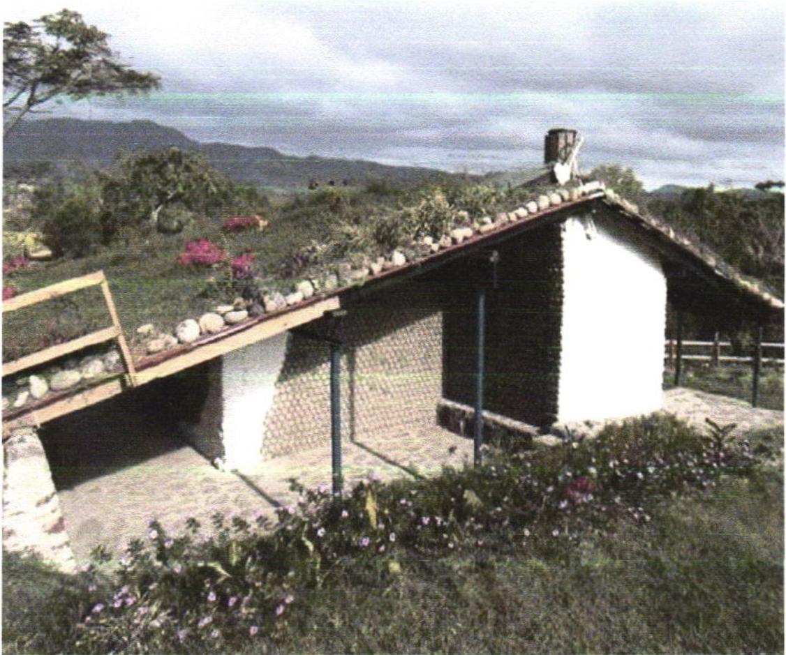
Figure 3.1.1. First house built with plastic bottles
