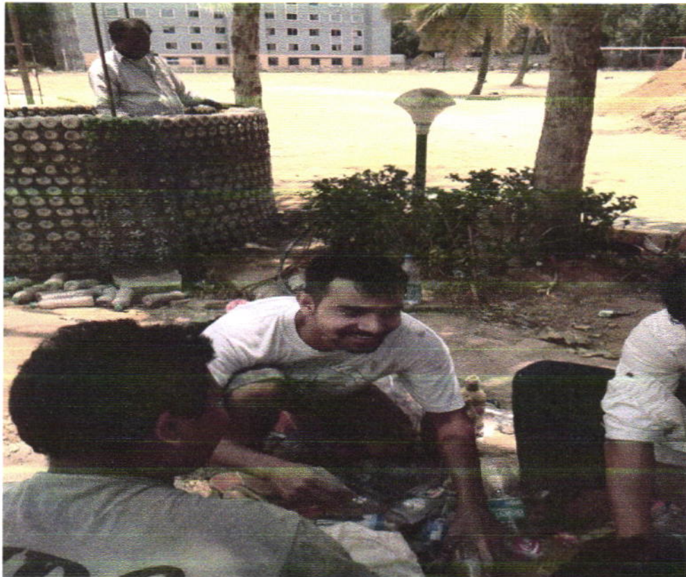
Fig 7.2.2: Filling the bottles with sand
