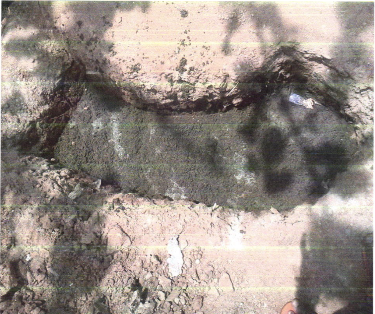
Fig 7.4.1: Concrete Bed
